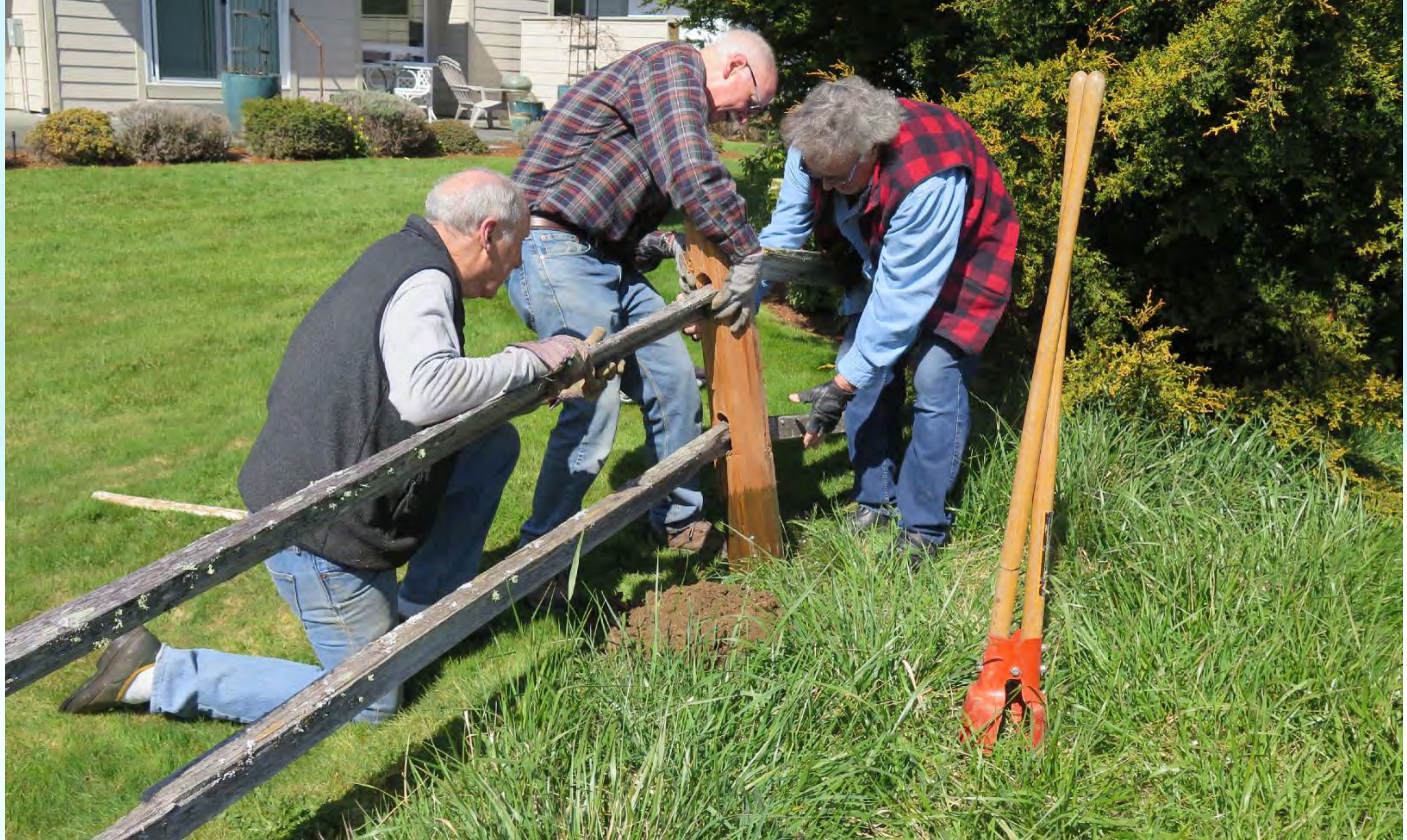
Fence post team replacing rotting posts and rails
