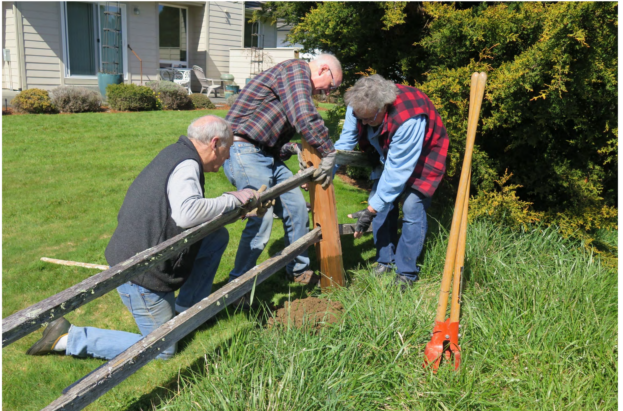
Periodic “Ad hoc” committee: Fritz Field, Doug Hale and John Meier replacing selected perimeter fence posts
